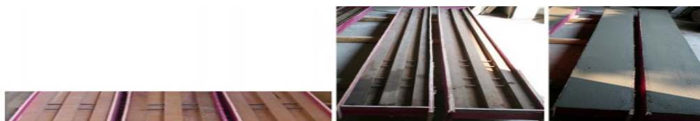
Figure. 5 Wood deck, steel connector, formwork, and finished beams [10]
